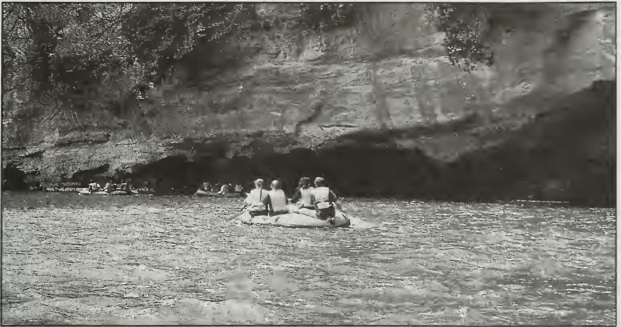
Figure 4-6. Photograph of undercut Vermilionville Sandstone at Mile 1.6.
